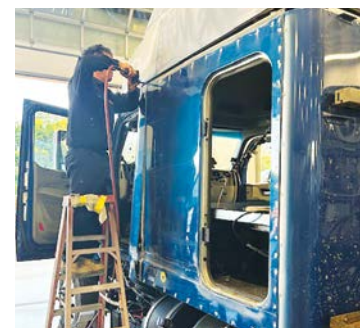
Located in Coon Rapids, MN, the Rihm Kenworth body shop focuses on fast, quality repairs.
