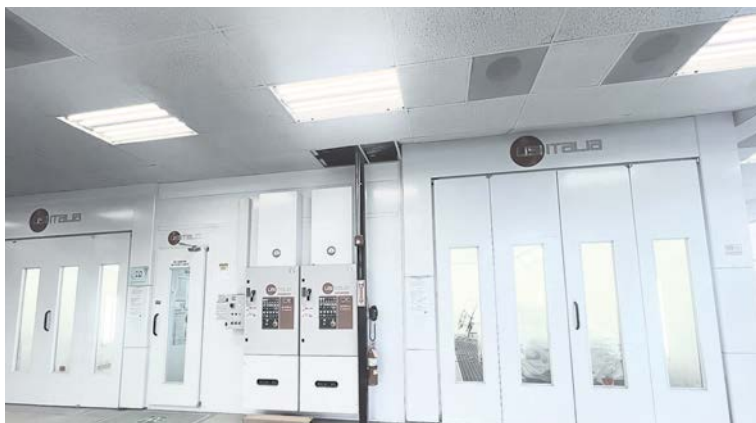
Moppert Brothers' Northfield, NJ, location was built to repair luxury cars, making the high-quality finishes produced by USI Italia booths a must.
